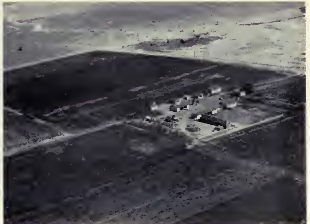
SPRINKLERS FOR SANDY SOIL. —The Winchester Development Form of the Columbia Basin project, Wash., was prepared for sprinkler irrigation because of the sandy nature of the land. Photos at left and right by H. E. Foss, Region 1.
